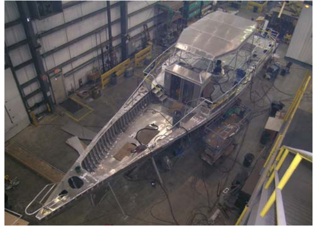
Figure 19 BLB-70 Hull Fabrication in Connecticut
